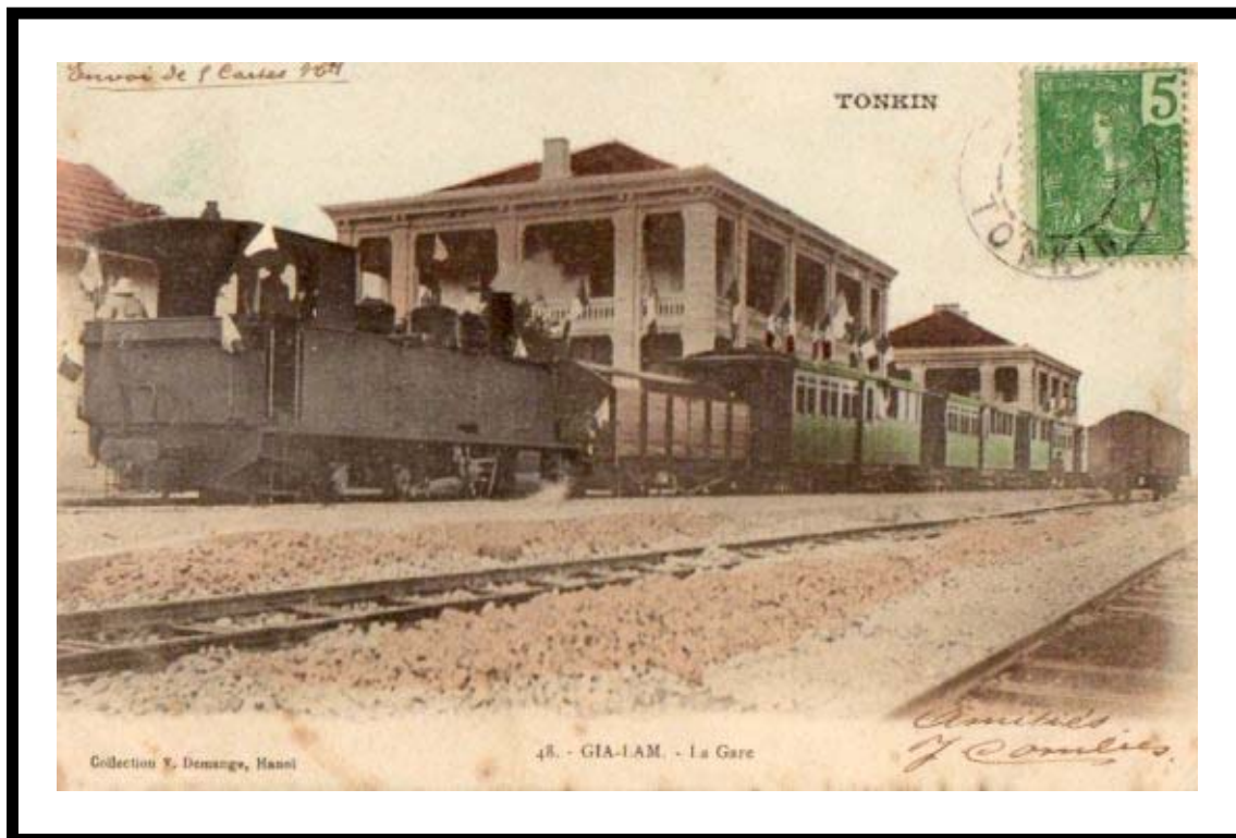
Gia-Lam Train Station
