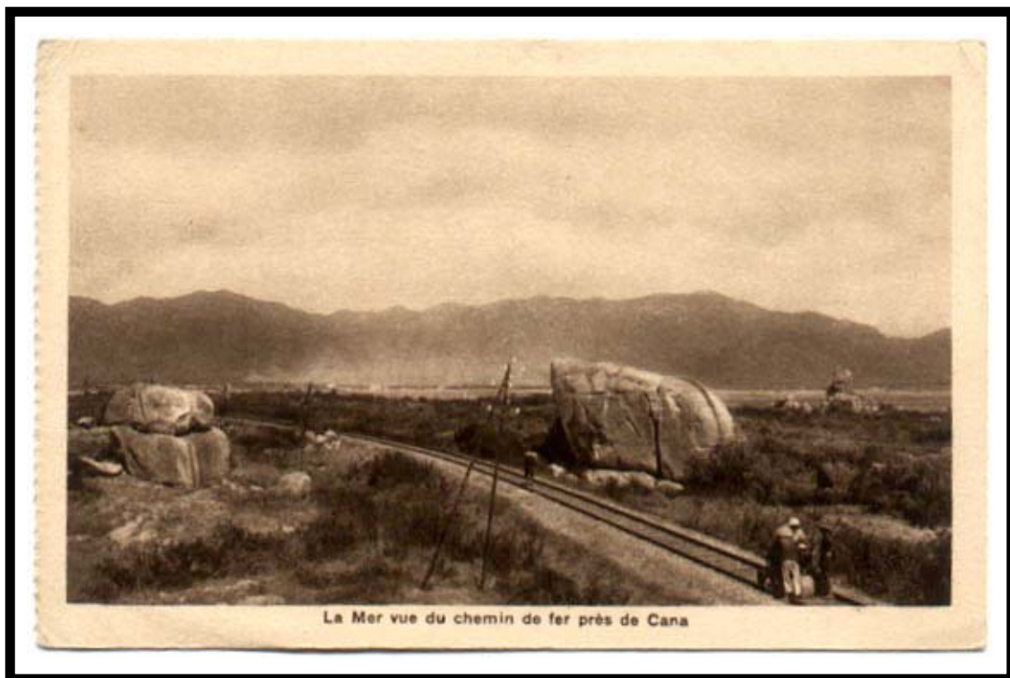
Panoramic view where the rail line approaches the sea near Cana, Annam.
